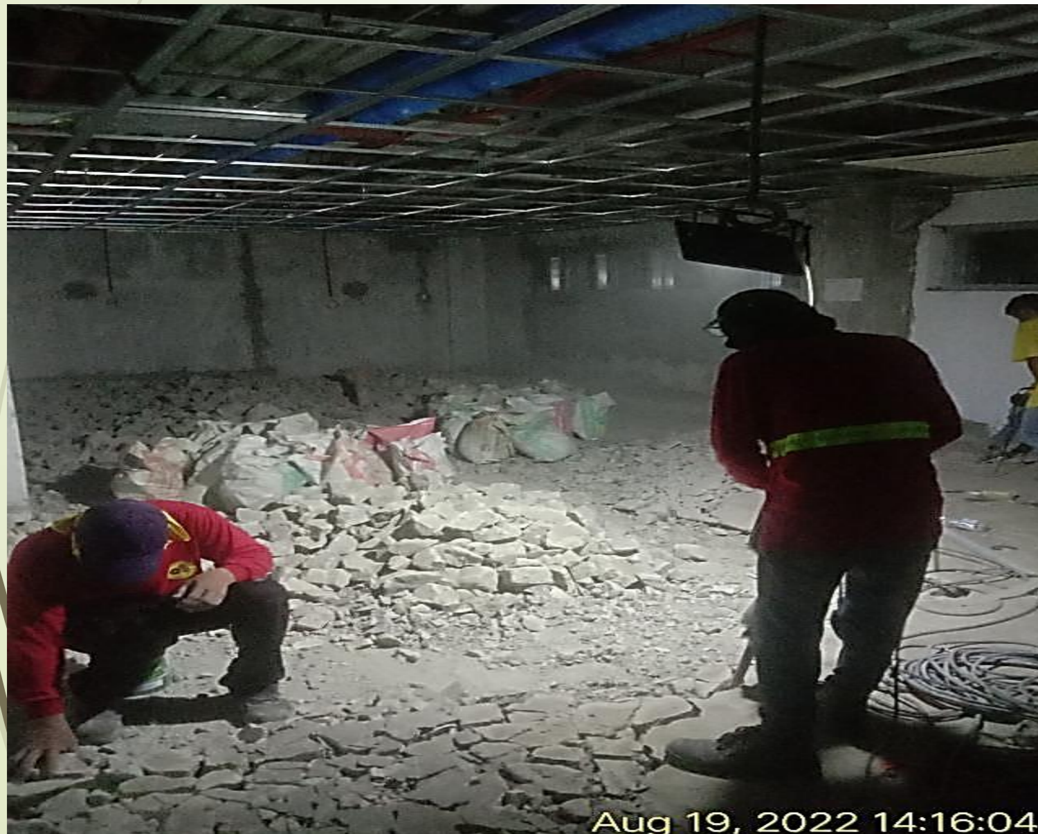
Chipping off of Concrete Floor..
