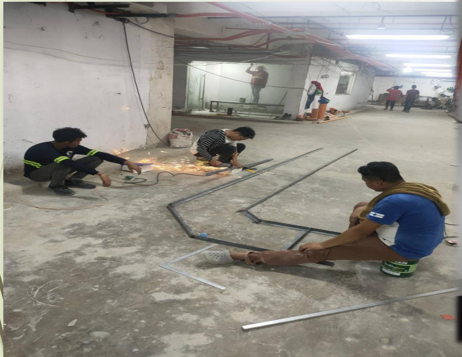
Fabrication of Cable Trays
